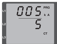
Fig. Current transformer programming mode The primary and secondary currents can be changed using buttons 1 and 2 (cf. page 52).
