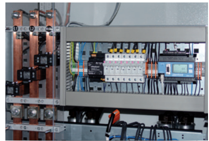
Fig.: Capacitor monitoring in a PFC system
