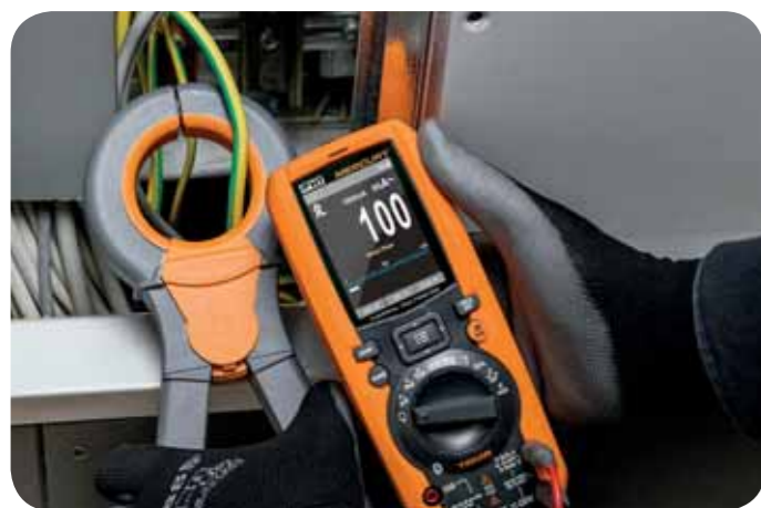
AC leakage measurement.
